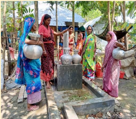
Photo: Collect Water from a Tap stand of the PWSS
